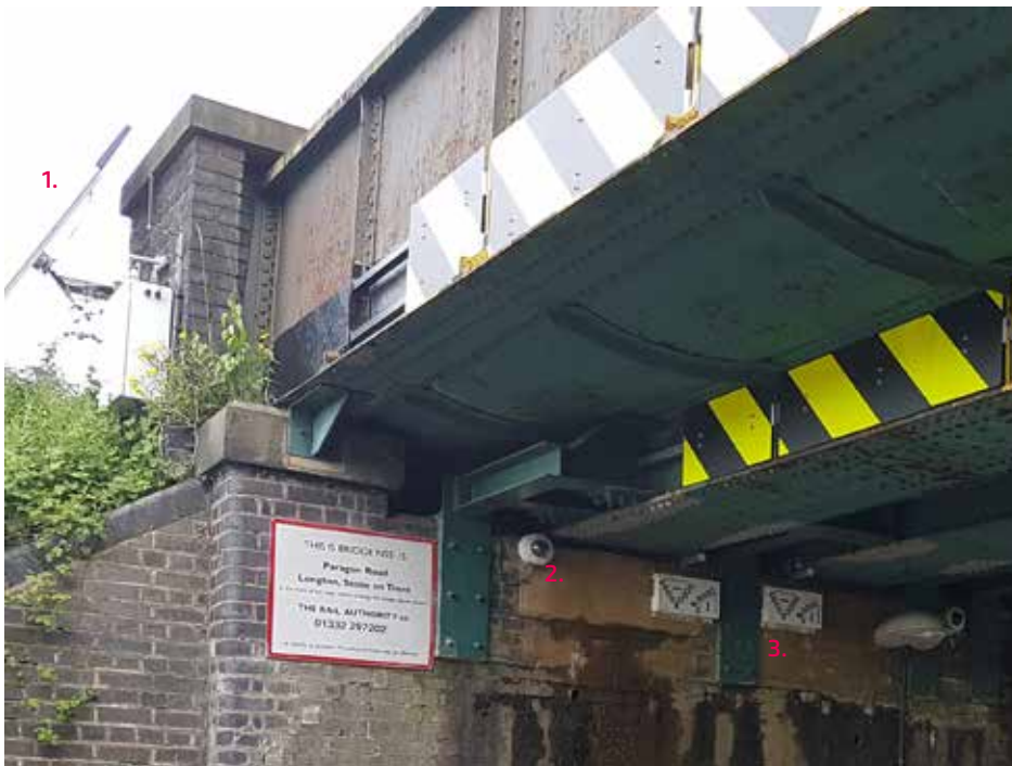
1. Solar Panel and Control Unit
