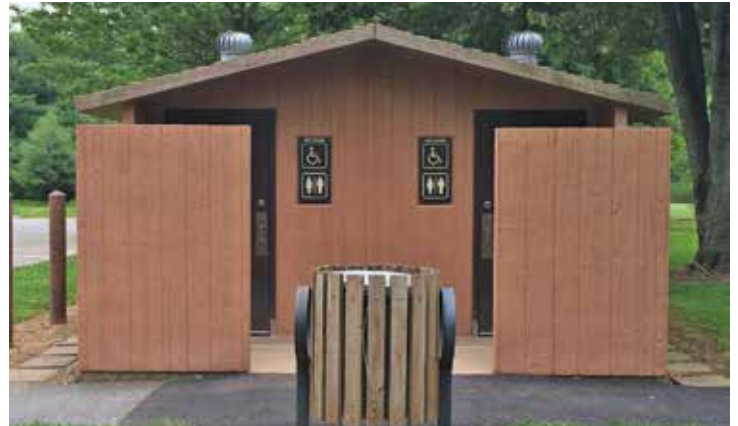
Custom screen for double vault restroom
