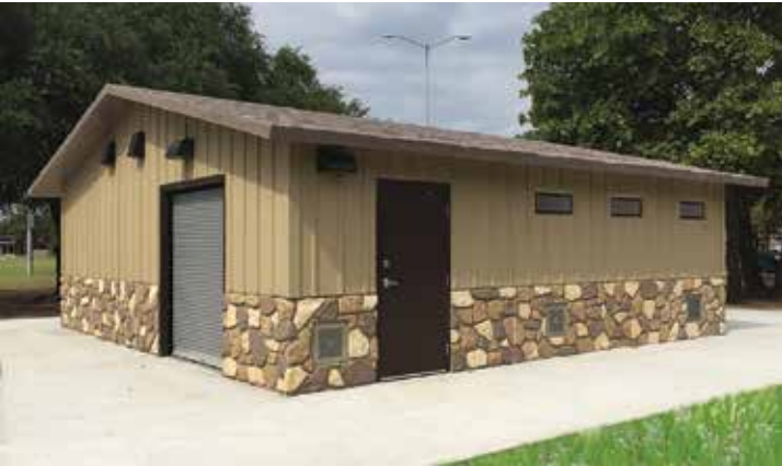
Flush restroom/concession with custom roll up door
