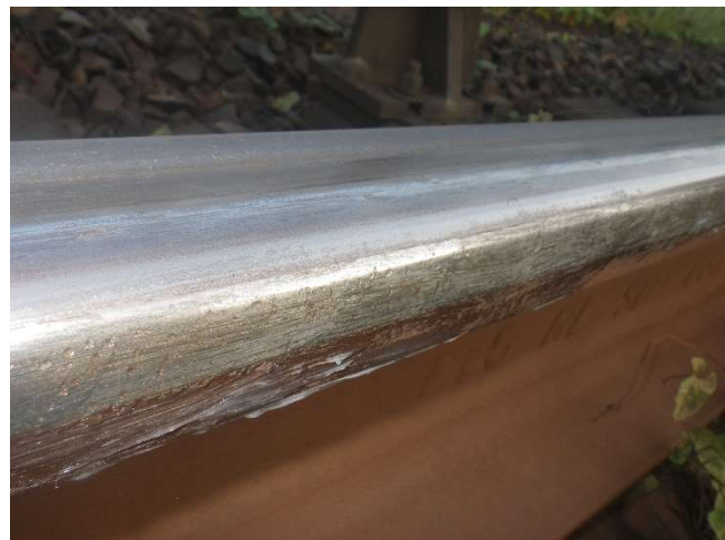
Figure 6. SYNCURVE™ Transit application using a paint guide (left) so that the grease was only applied to the gage corner and gage face (right).
