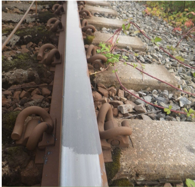
Figure 5. KELTRACK® Trackside Transit applied to the rail.
